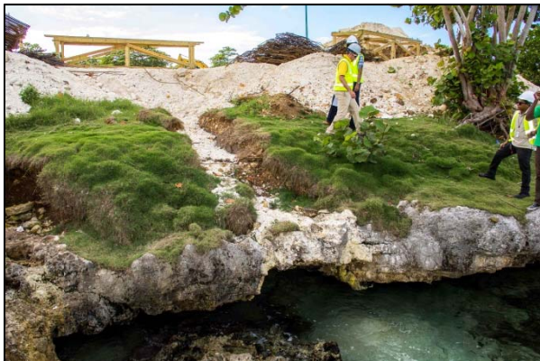
Photo 3. Section of the property showing runoff carried down into the marine environment. There is no berm in place or sediment trap. (Photo taken by NEPA Officer on 17 December 2015)
