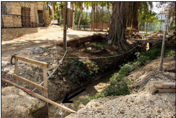
Photo 2. Section of the main drain to show that sediments and runoff from the site can easily get into the drain and into the marine environment. Black arrow shows sediment n drain. (Photo taken by NEPA Officer on 17 December 2015)
