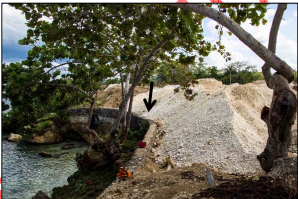
Photo 4. Inadequate berming of storage material. Black arrow shows where there is overspill to the marine environment. (Photo taken by NEPA Officer on 17 December 2015)
