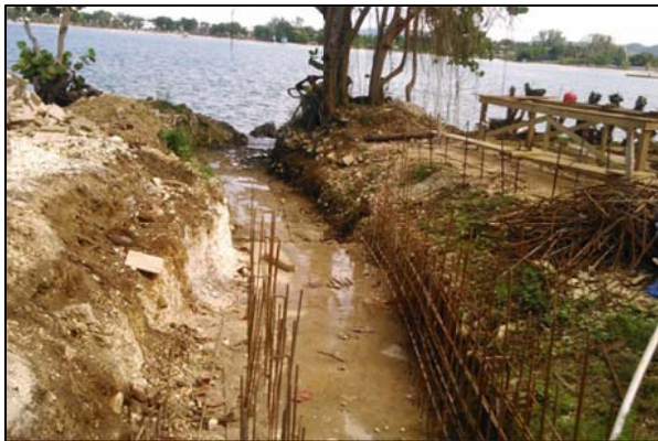
Photo 1. Box culvert under construction in the main existing drain on property. Also note that there is no sediment trap where the drain exits to the sea. (Photo taken by NEPA Officer on 11 December 2015)
