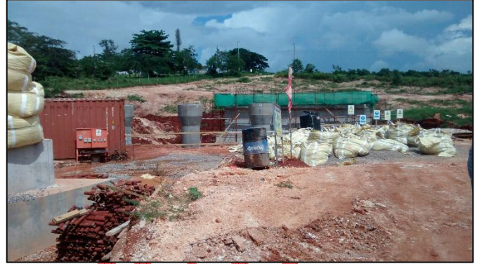
Photo 2: Bridge under construction. (Photo taken by Environmental Officer, NEPA on 28 October 2014)
